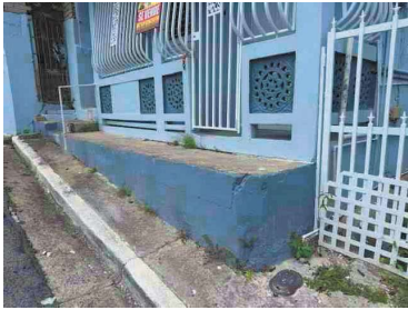
Install Security Railings
