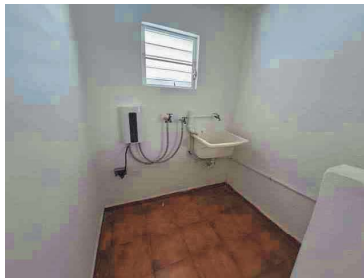
Laundry Area - Unit #2
