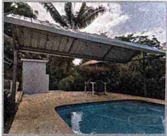
Roof Over Pool
