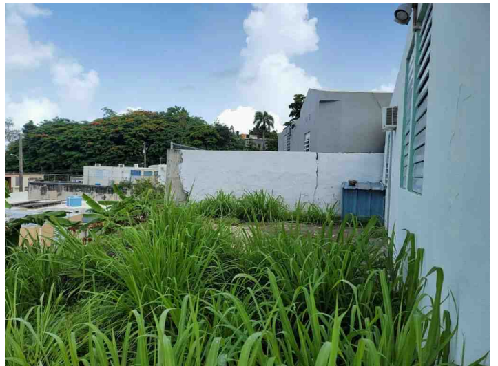
Install safety fences at its adjoining point
