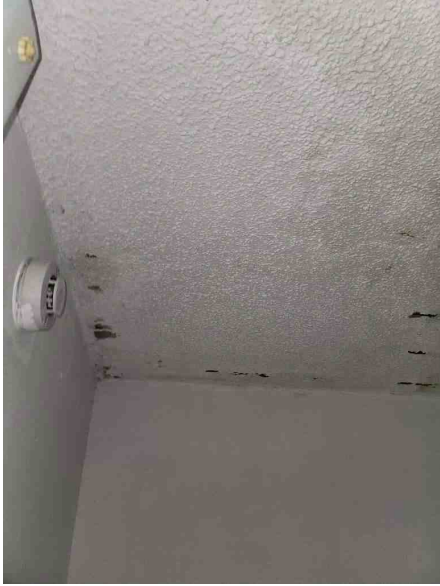
Repair & Paint all interior ceiling
