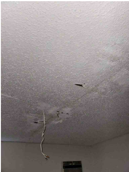
Repair & Paint all interior ceiling
