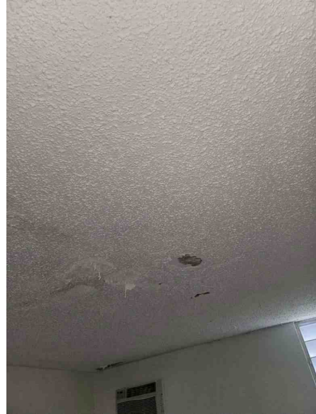
Repair & Paint all interior ceiling
