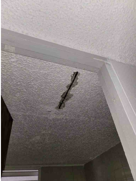
Repair & Paint all interior ceiling
