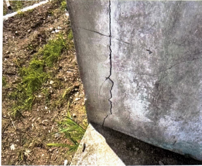
Wall Crack
